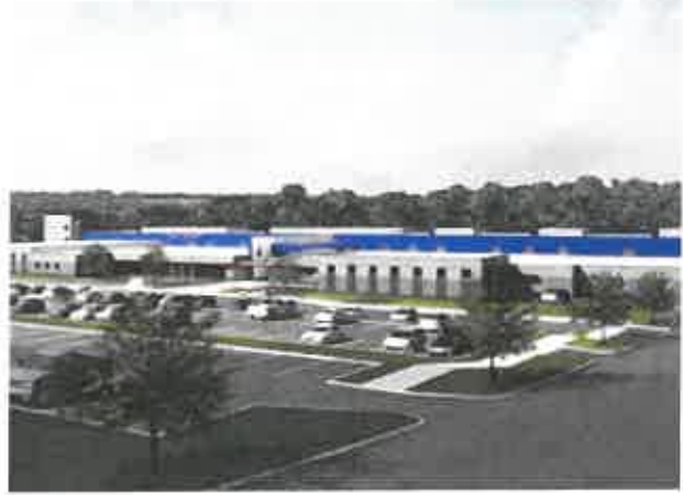
Howard County, MD New Detention Center Jessup, MD
