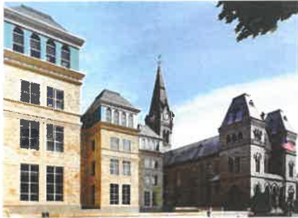
Blair County, PA Courthouse Renovations/Additions Hollidaysburg, PA
