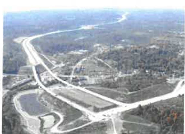
Pennsylvania Turnpike Commission Mon/Fayette Expressway Pennsylvania
