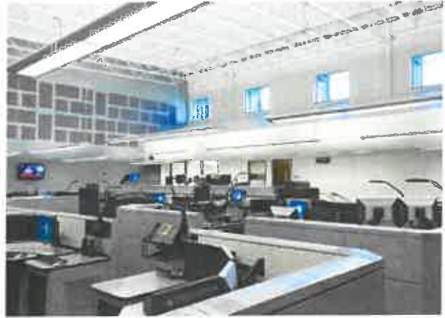
York County, PA Emergency Services / 911 Center York, PA
